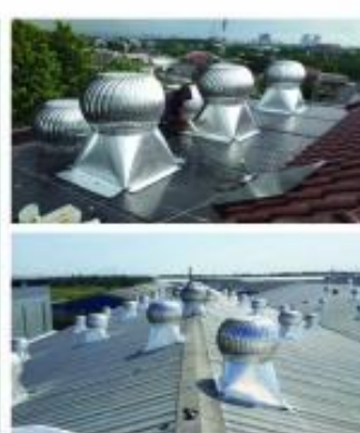
CYCLEVENT TURBINE VENTILATOR NON ELECTRIC TYPE CV-105 Bahan : Aluminium & Stainless Steel 430/304 Bearing : SKF Full Stainless Steel, Made In Japan Diameter : 105 CM = 42" Dimensi : 347 x 154 x 154" Berat : 20.5 kg / 25 kg Kapasitas Hisap : 5940 M 3 / menit
